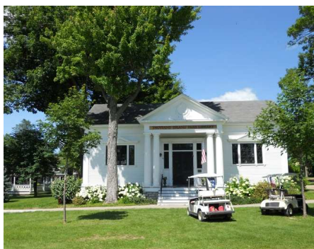
Library exterior, with golf carts (TI Park residents' preferred mode of transportation) parked out front
