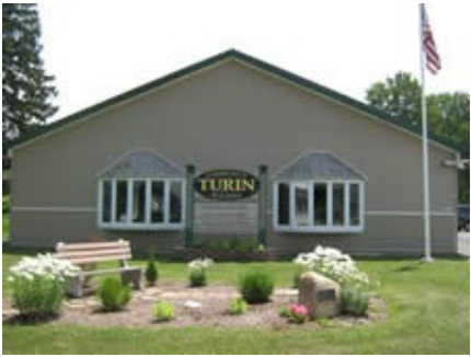
Front of building
